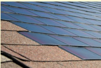
Amorphous thin film solar cells
