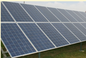
Multicrystalline or polycrystalline solar cells
